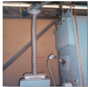
Boiler Auger
