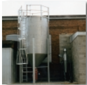
Three-Ton Pellet Hopper
